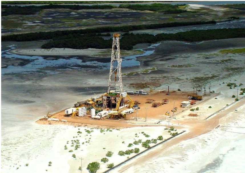
Fig. 1. Workover rig performing a maintenance service
